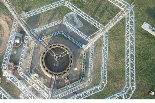
WASProject, Big Delta 3D printer for adobe houses, 3D printer, additive manufacturing, adobe and fluid-dense materials Photo credits: WASProject
